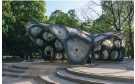
Elytra Research Pavillon, pavillon en fibre de carbone © ICD/ITKE University of Stuttgart
