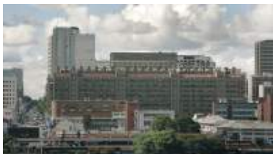
Vue d'ensemble de l' Eastgate building © Mick Pearce
